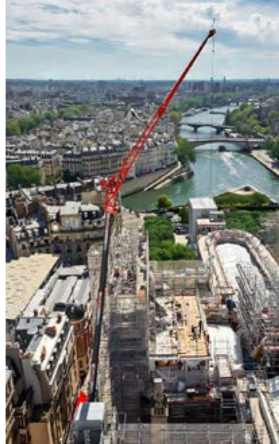
At the very edge of the building The LTM 1120-4.1 extends far beyond the nave. With its 19-metre-long, hydraulically adjustable double folding jib on the telescopic boom, the crane is able to transport its loads over long distances despite being positioned by the cathedral wall.
