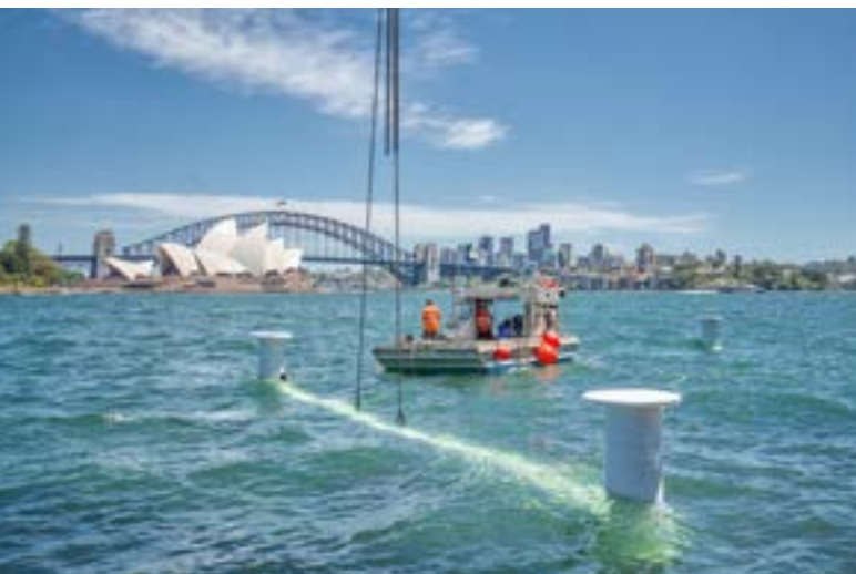
The divers and crane drivers are a well-rehearsed team.
