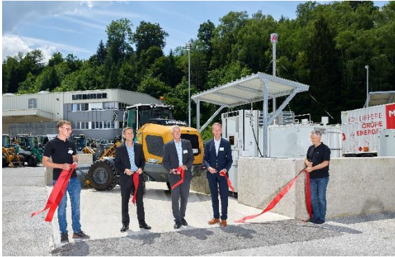
liebherr-L566-H2-Event-Bischofshofen-inauguration-06-2024.jpg The hydrogen refuelling station was officially opened at the plant site in Bischofshofen.
