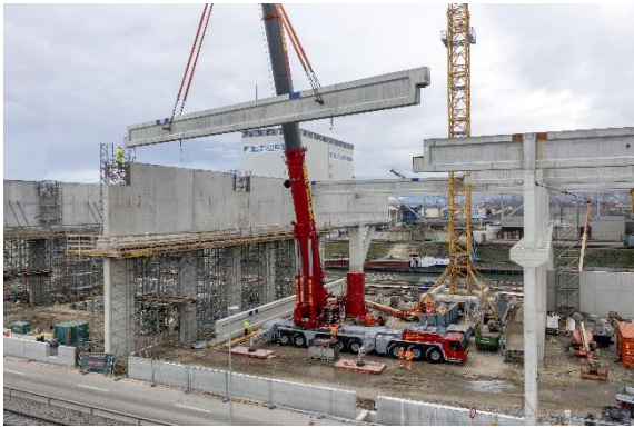
liebherr-ltm-1650-8-1-egger-3.jpg Closing the gaps: the LTM 1650-8.1 installed the last bone girders.
