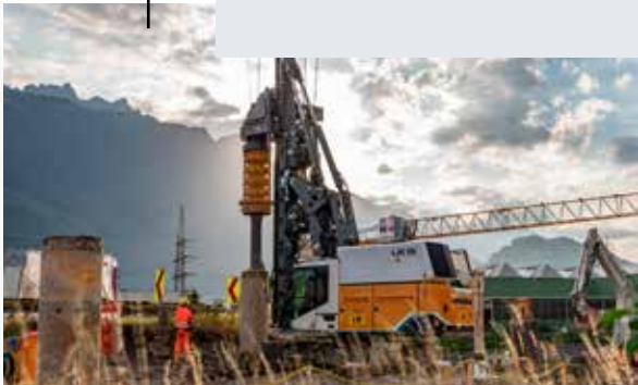
All quiet on the building site: Liebherr opens a new chapter with the LB 16 unplugged.
