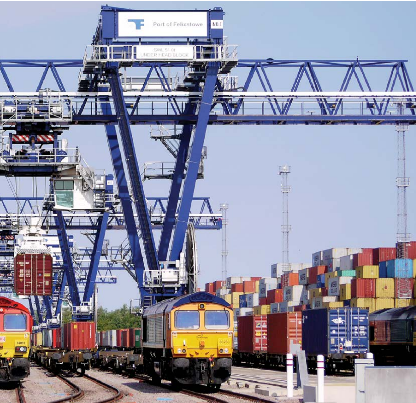
Rail mounted gantry cranes, Felixstowe, UK
