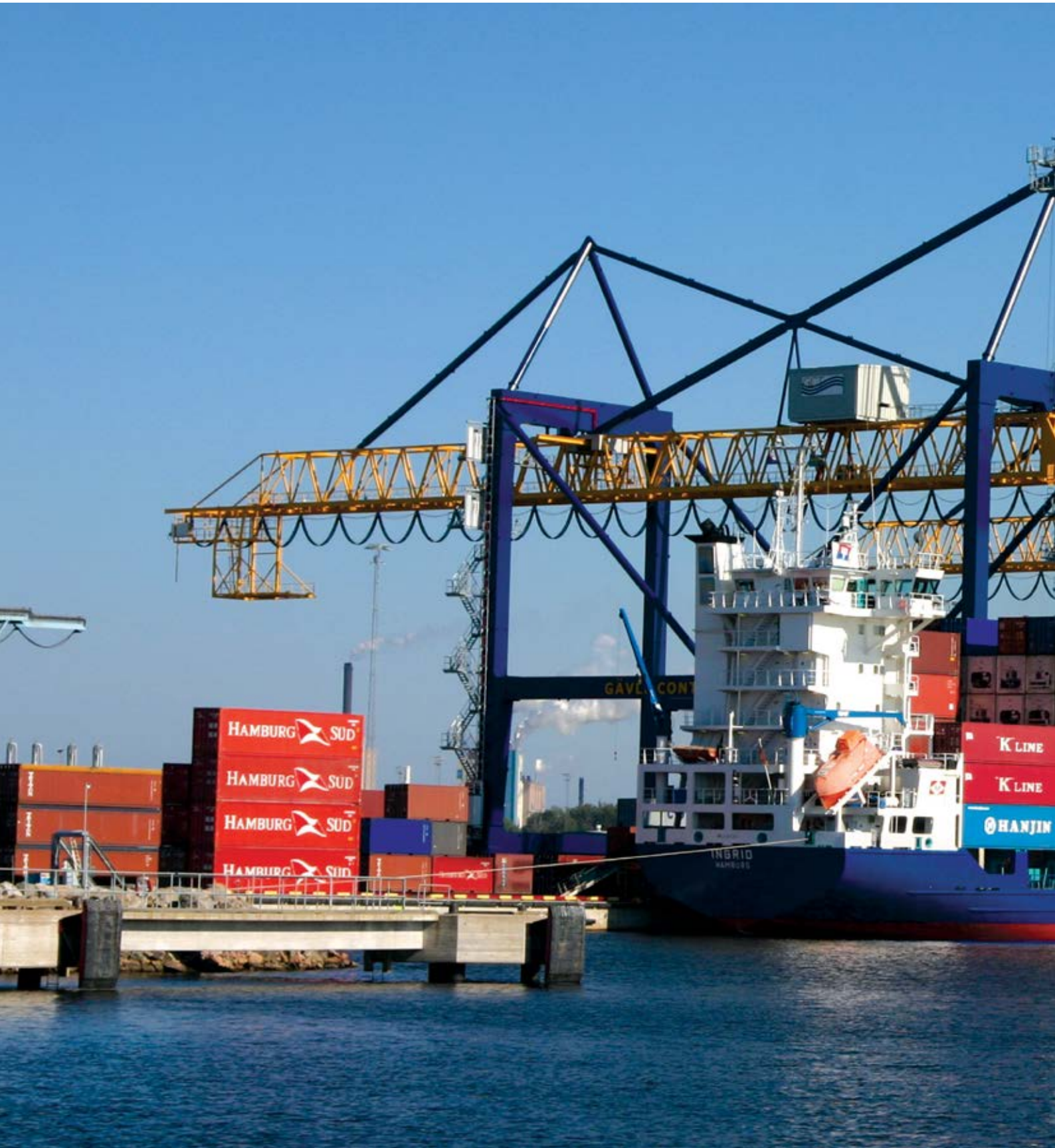
Wide span ship to shore stacking cranes, Gavle Container Terminal, Sweden
