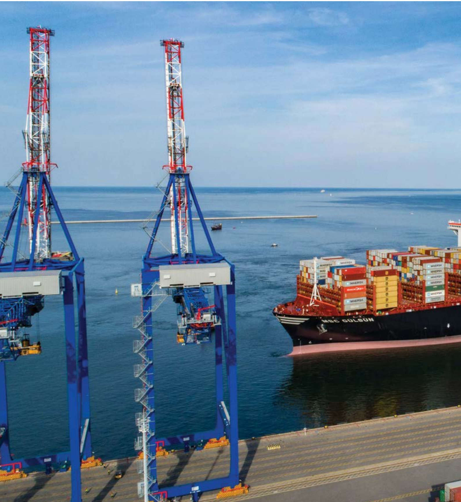
Megamax ship to shore cranes, DCT Gdansk, Poland
