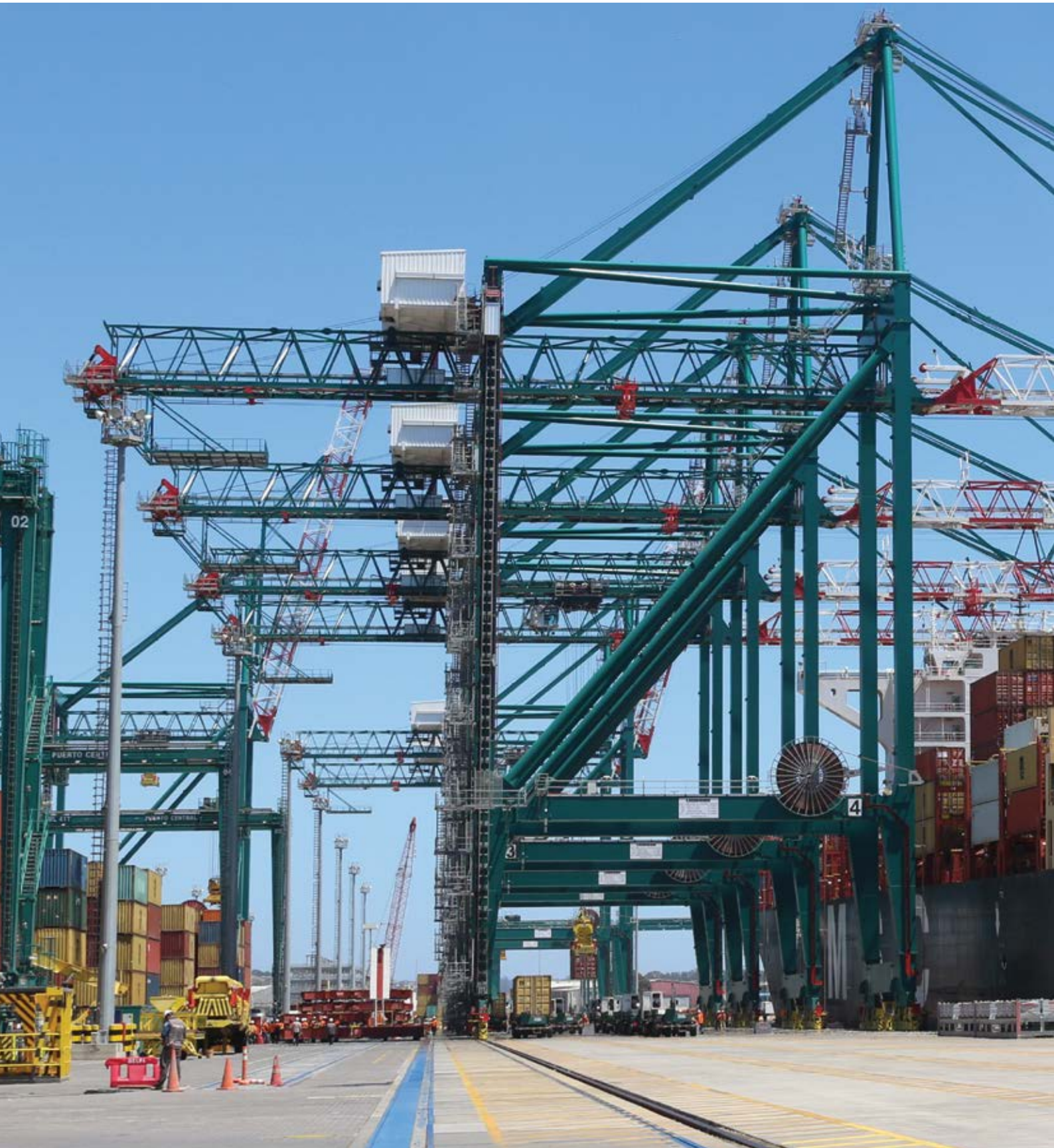
Super post panamax ship to shore cranes, Puerto Central, San Antonio, Chile
