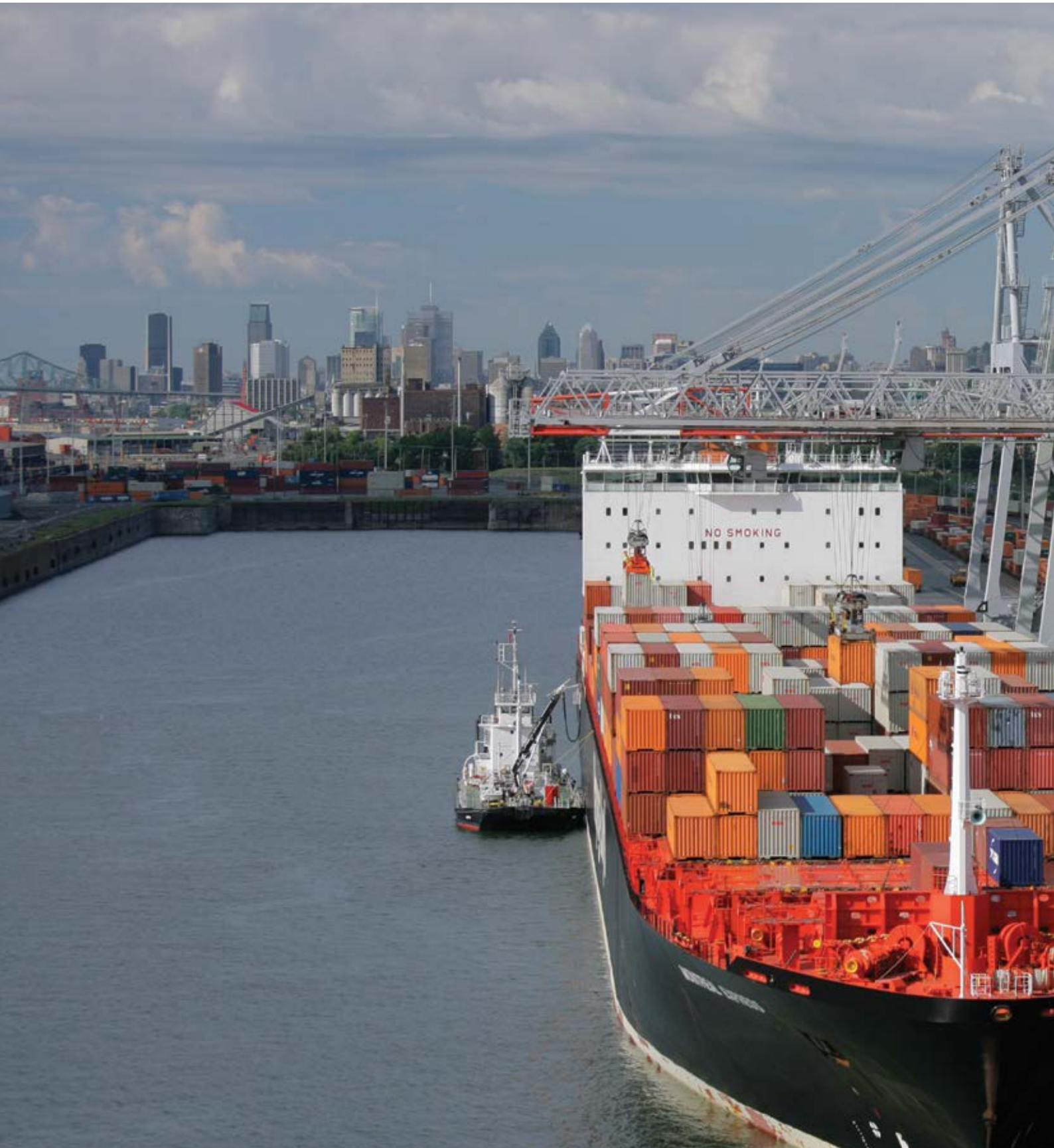
Panamax ship to shore cranes, Racine Terminal, Port of Montreal, Canada
