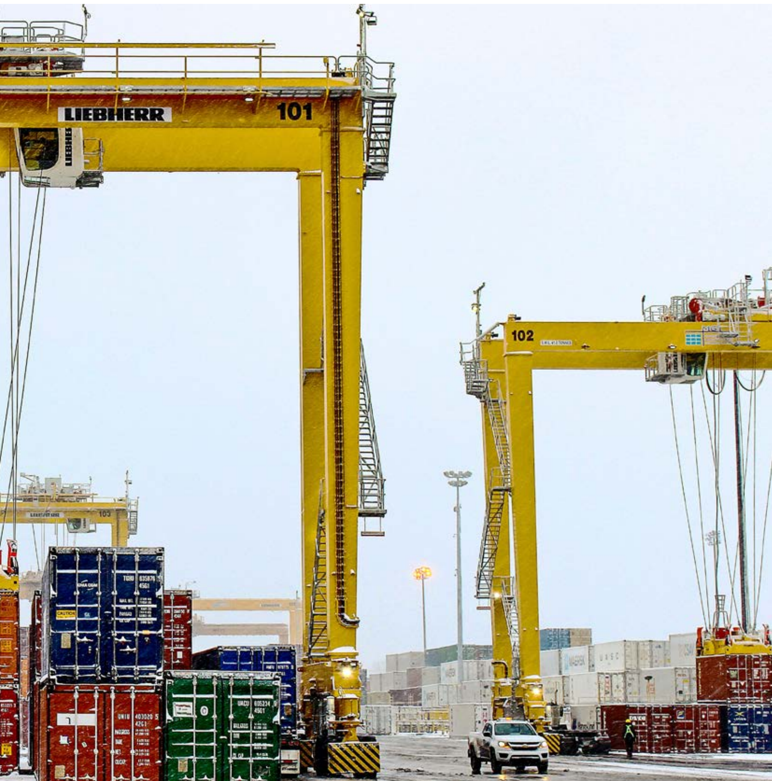
Rubber tyre gantry cranes, Montreal Gateway Terminal, Canada
