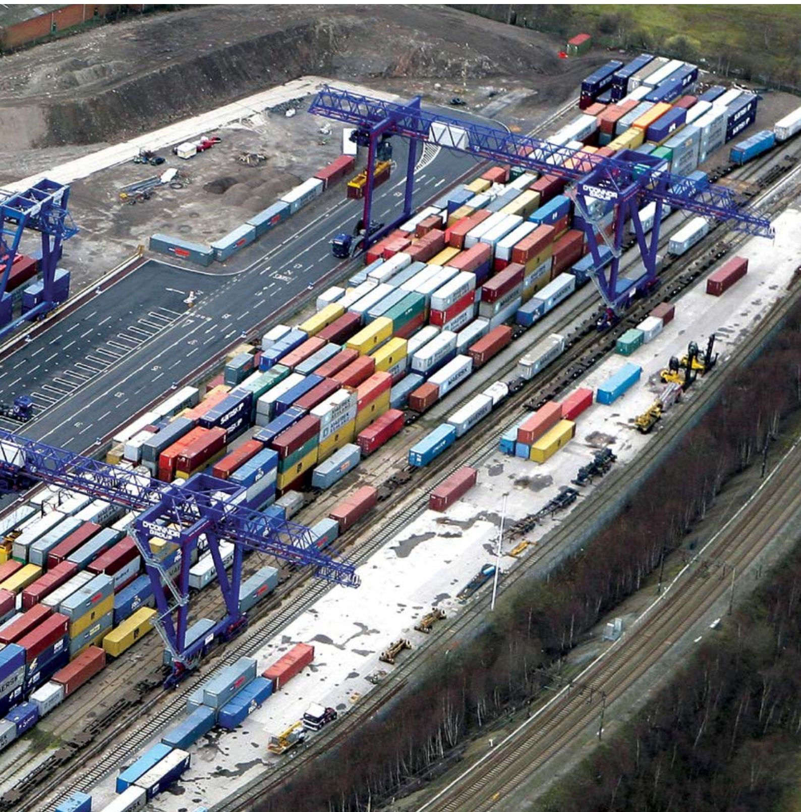
Rail mounted gantry cranes, stobart Group, Widnes, UK
